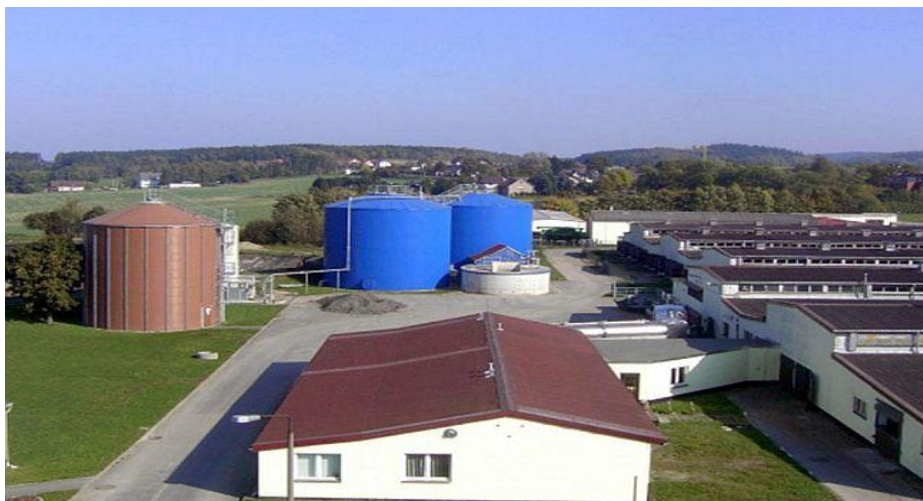
Figure 5. Anaerobic digestion plant.
